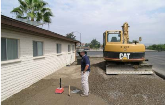
Figure-8: Density Testing of Aggregate Base
