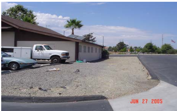
Figure-5: Fire Truck Wash Area – Before
