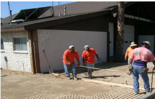
Figure-10: Mat Installation
