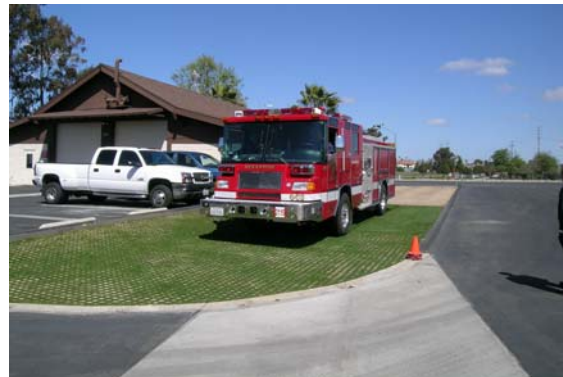
Figure-6: Fire Truck Wash Area - After
