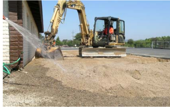
Figure-9: Placement of sand/organic layer
